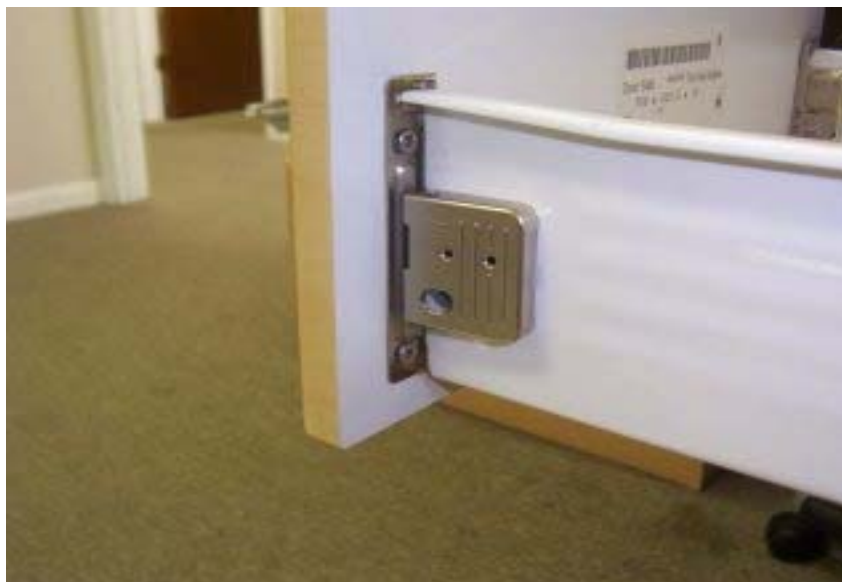
With your fingers, just push the clip to close and secure the front to the drawer box assembly.
