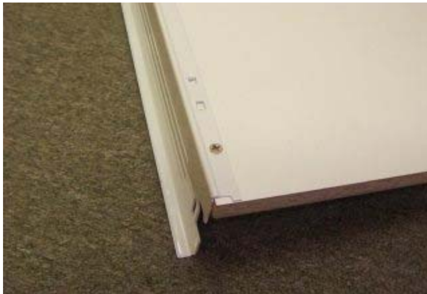
Place euro screw in front hole to secure the bottom
